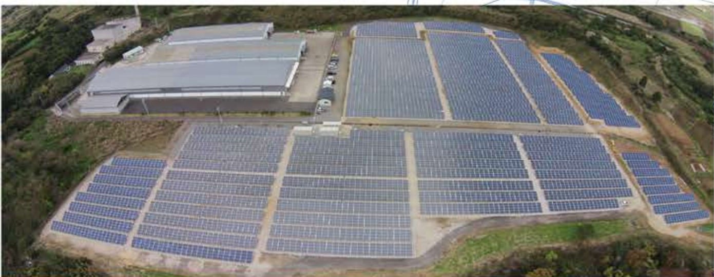
Fukuoka, China 2MW Ground Plant
