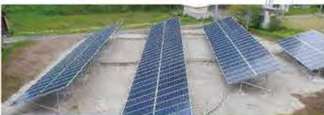
Hefei, China 54kW Rooftop Plant
