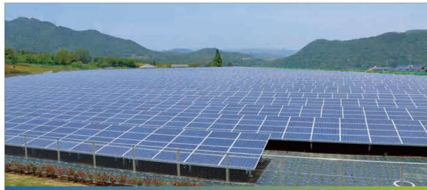
Gunma, Japan 1MW Ground Plant
