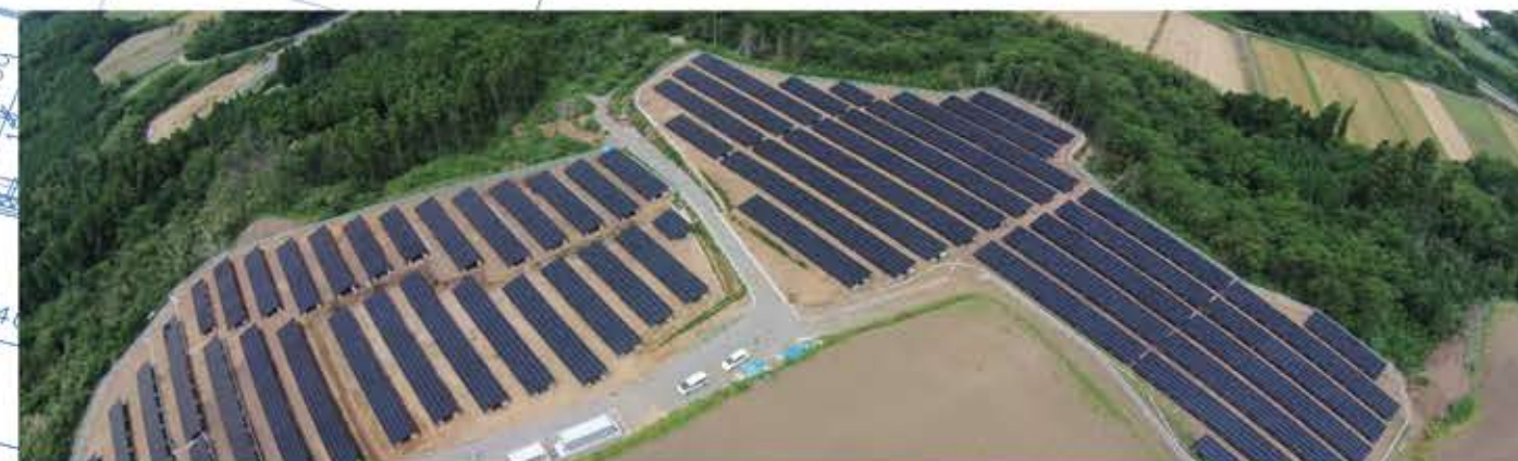
Minamishima, Japan 1MW Ground Plant
